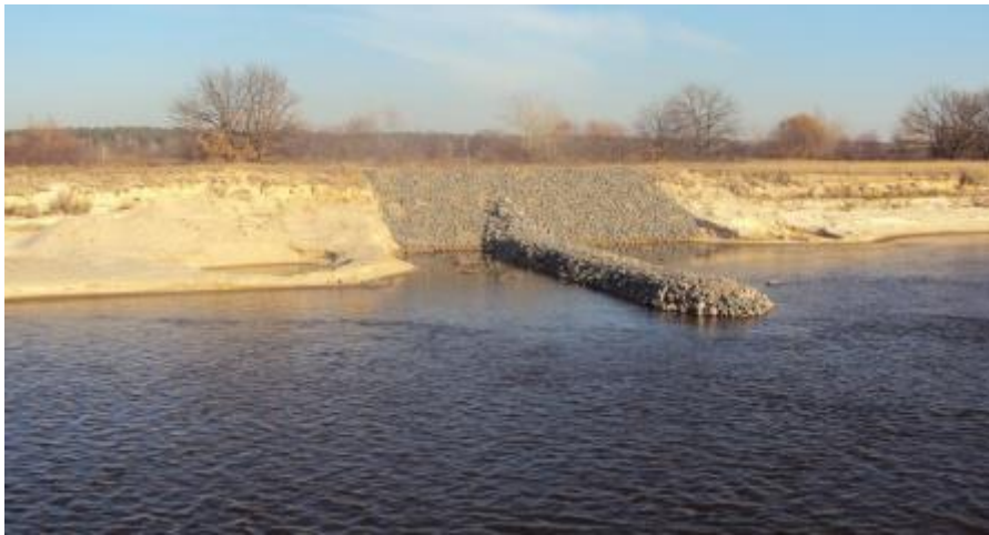
Fig. 25. Example of a side-spur on the Pripyat river
